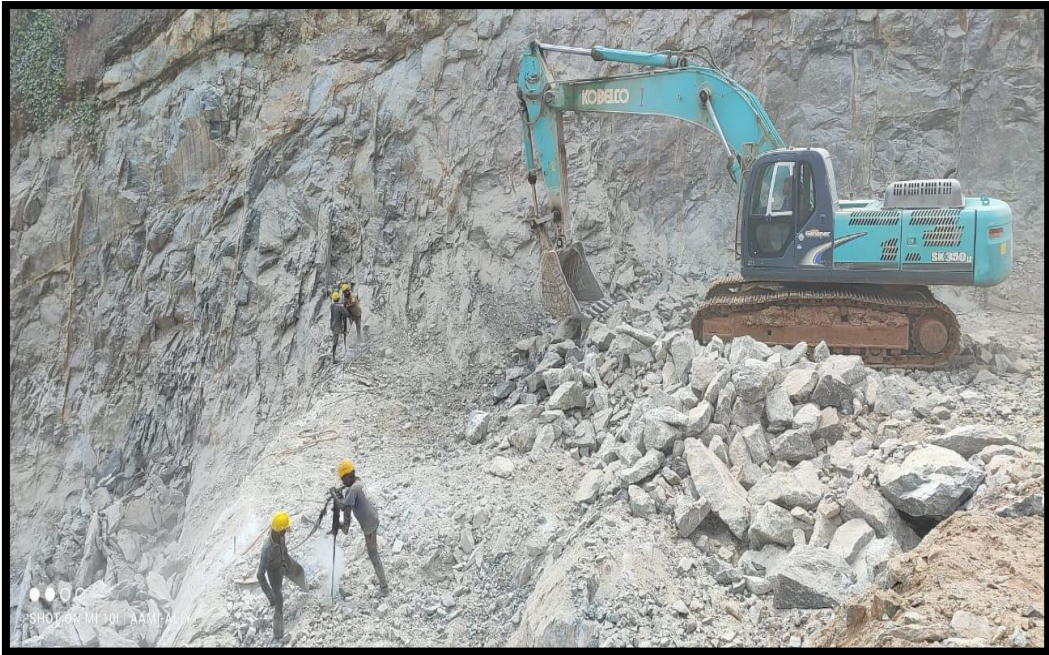
Workers with personal protective equipments
