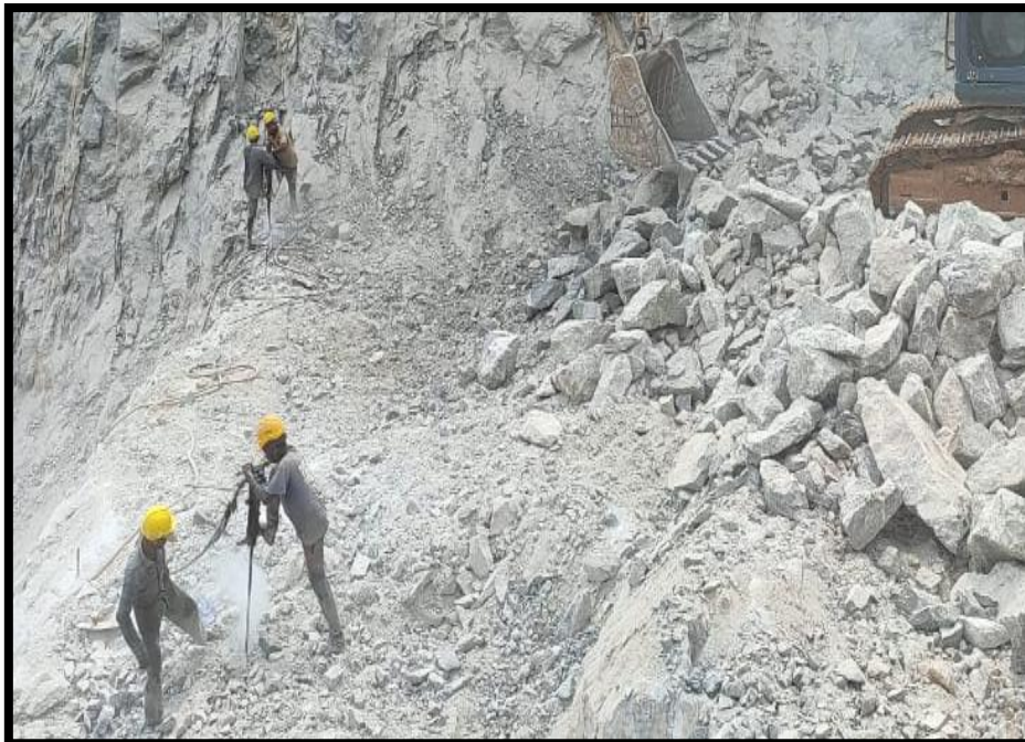
Workers with personal protective equipments
