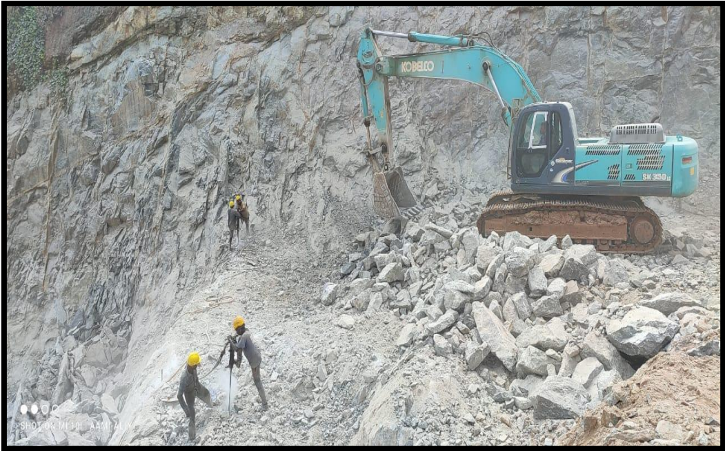
Workers with personal protective equipments
